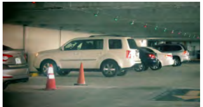
Single space sensors monitoring space availability.
