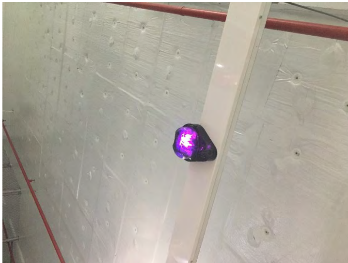
Figure 15: TUS-300 Uni-Strut/Rail mounting
