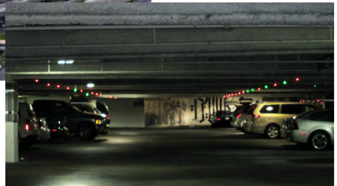
Ultrasonic single space sensors monitor every parking space.
