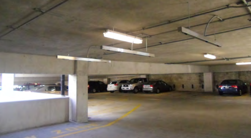
Custom entry sign and ultrasonic directional sensors at garage/level entry/exit.
